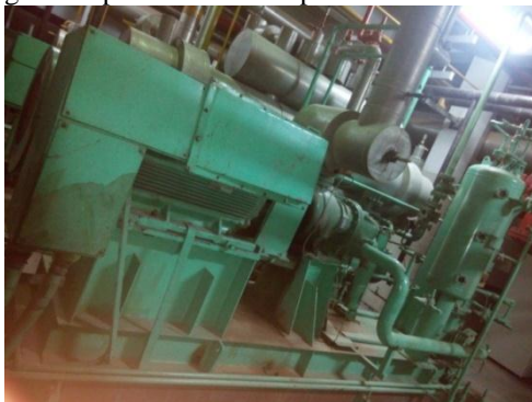
Fig 3.2 Refrigeration Unit of BAMUL
